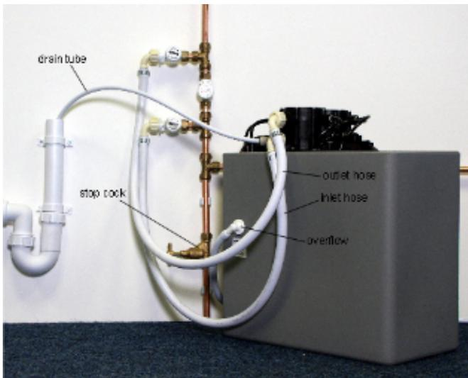
4. Turn off the inlet, outlet and bypass valves.
