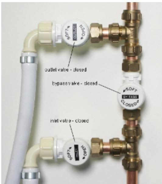
5. The drinking water tap connection and the garden tap connection should be made in the pipe between the stopcock and the bypass valve.
